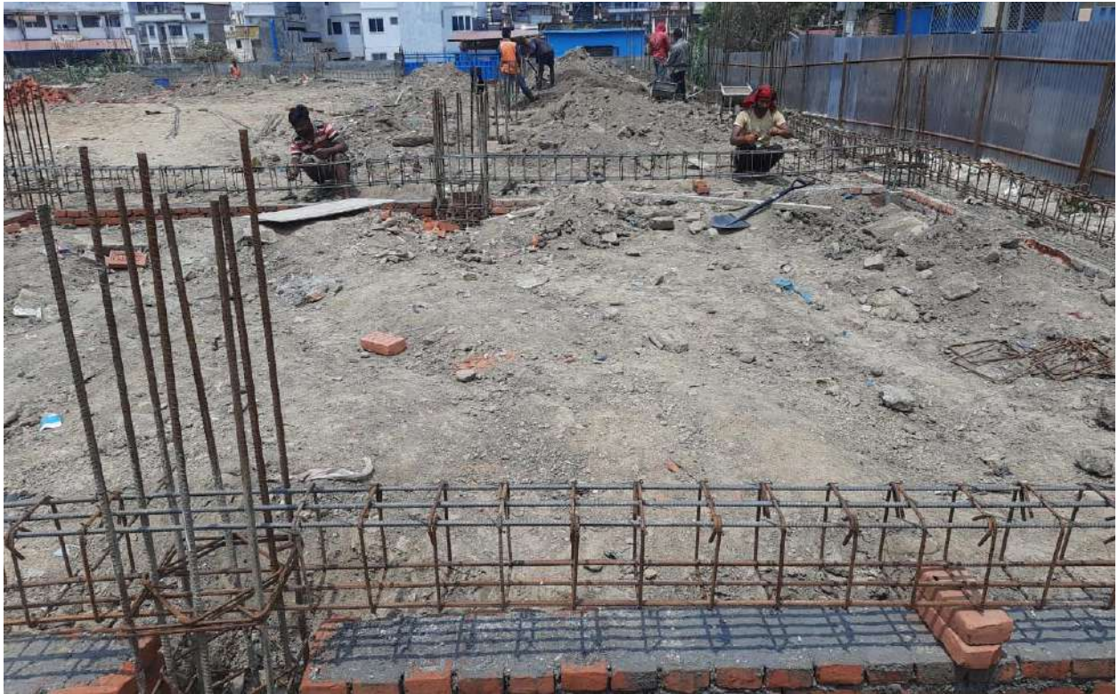
TIE BEAM REBAR WORKS
